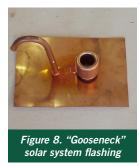
having jurisdiction, or in the absence of such code, the latest version of the IRC and IMC (See IRC M2301.2.9, IMC 1402.7.2). Figure 8 shows a "gooseneck" flashing that is commonly used for solar thermal installations to seal both piping and electrical penetrations.
