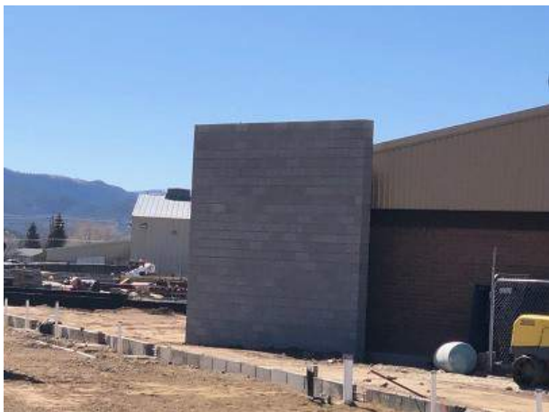
Temporary fire wall
