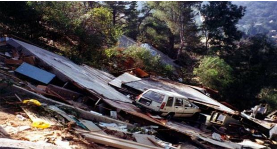
Figure 4. Hillside dwelling collapsed in the 1994 Northridge, California Earthquake (Credit: City of Los Angeles Department of Building and Safety).
